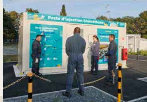
Biomethane injection station
